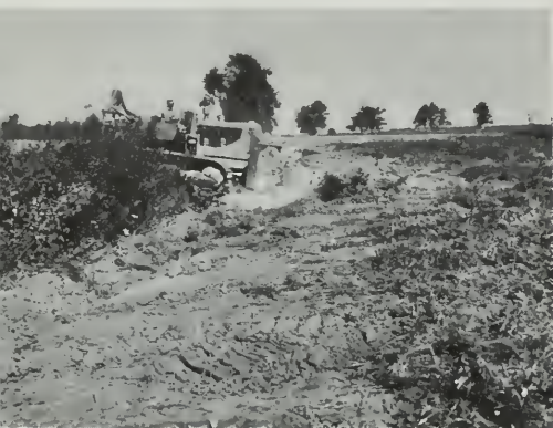
The gully was filled, and a waterway was developed.
